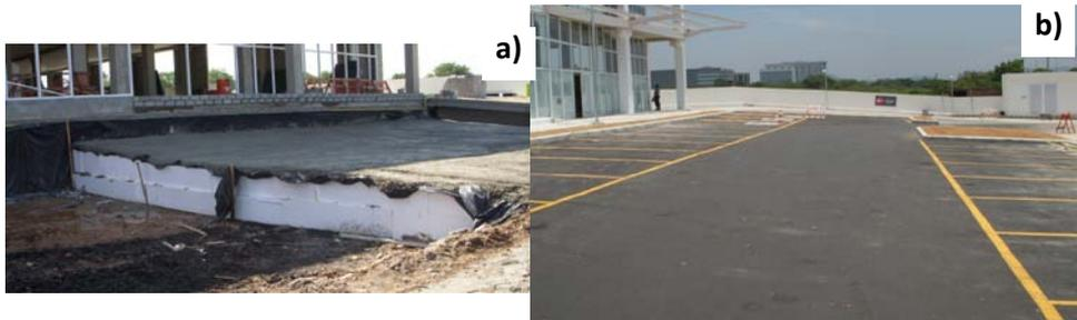
**FIGURE 9** Use of EPS blocks as lightweight fill material: a) cross section showing blocks and protective cover; b) finished pavement (Lima and Almeida 2009).
