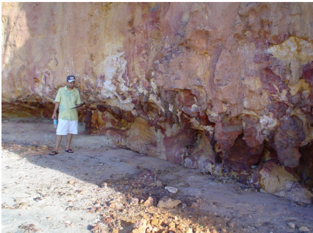
Figure 7. Erosion at the toe of the sea cliff caused by sea action in Central Section.
