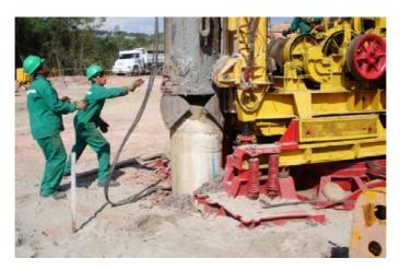
FIGURE 8. Finished geosynthetic encased sand column.
